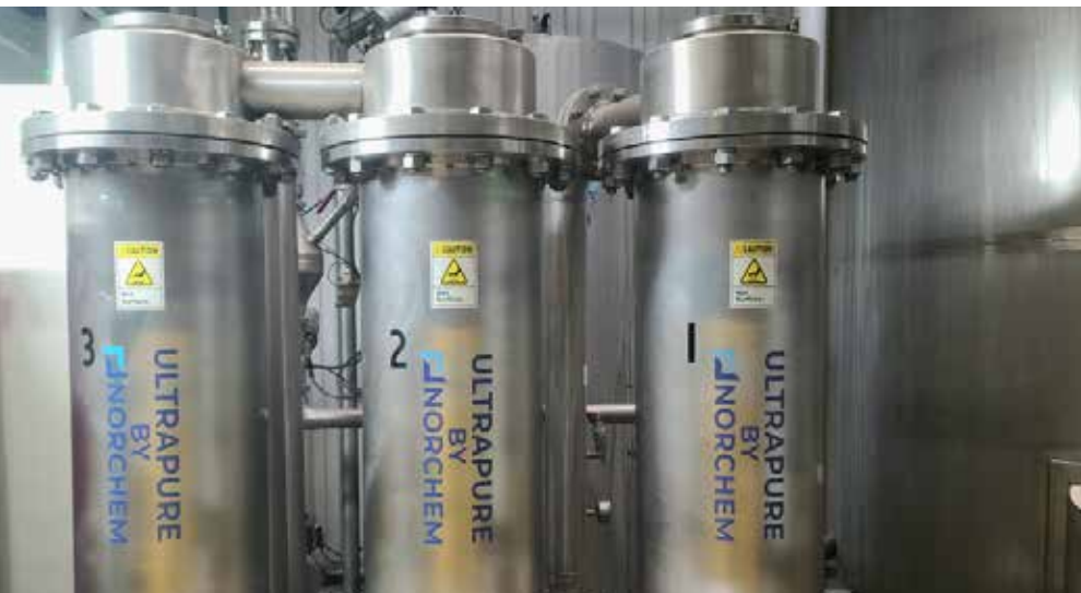
Above: A ceramic-filtration system for washwater at Mickey's Linen in Villa Park, IL. The three ceramic-membrane canisters can process 70–80 gallons per minute (GPM). The ceramic-filtration system for rinse water has two canisters that can process 40–50 GPM.
